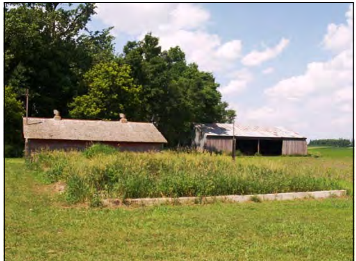
Subject property outbuildings.
