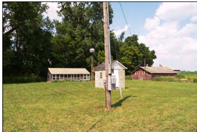
Subject property additional outbuildings.
